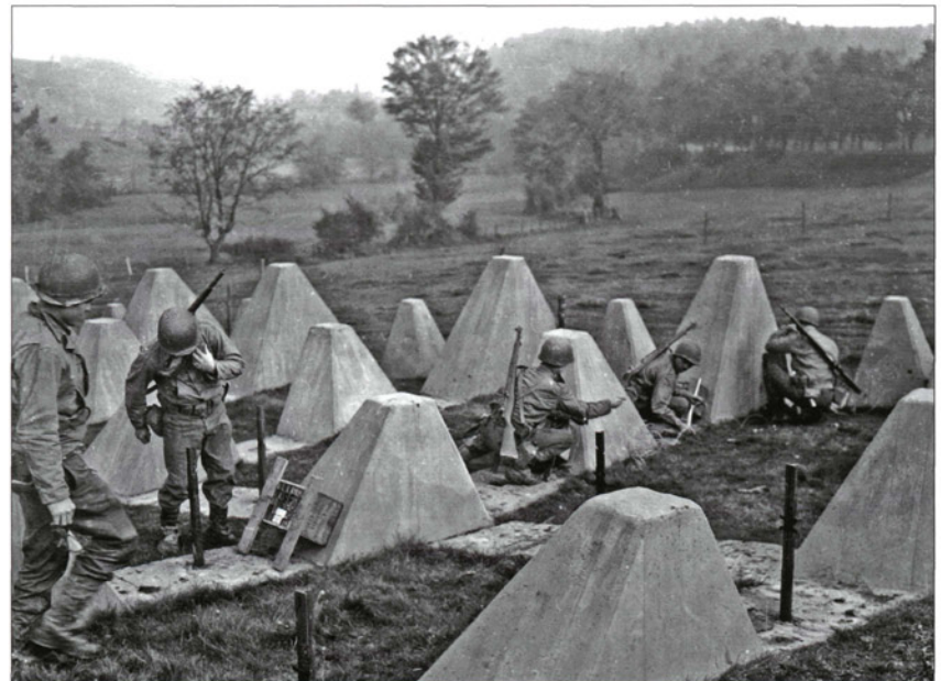
Engineers of the 3rd Armored Division plant demolition charges on dragon's teeth along the Scharnhorst Line in September, trying to blast another corridor towards Aachen. (NARA)
