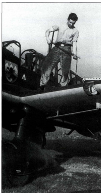
An armourer reloads the port 7.9 mm MG 17 wing machine gun of this aircraft of the Stabskette II./StG 77
